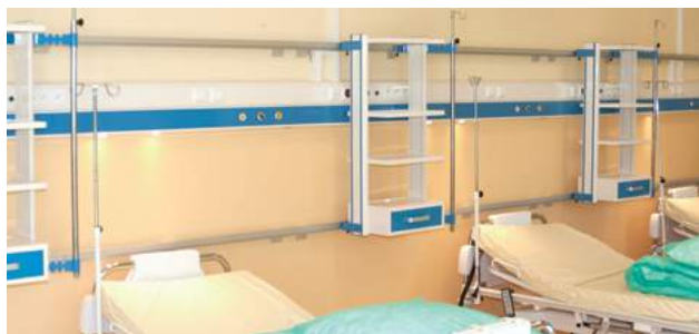
Sample solution of supply unit ISA 9000 with ISA system rail equipment - mounted directly to the wall
